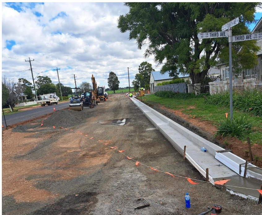
Figure 6: New Kerb and Gutter on Fourth Ave is nearly complete
