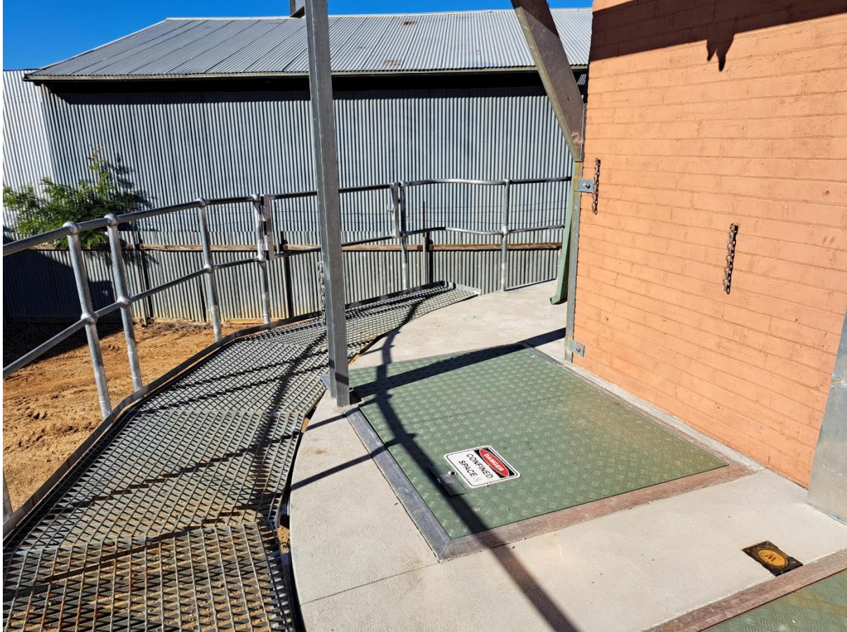
Figure 1: Narromine's main sewer pump station recently had safety works completed
