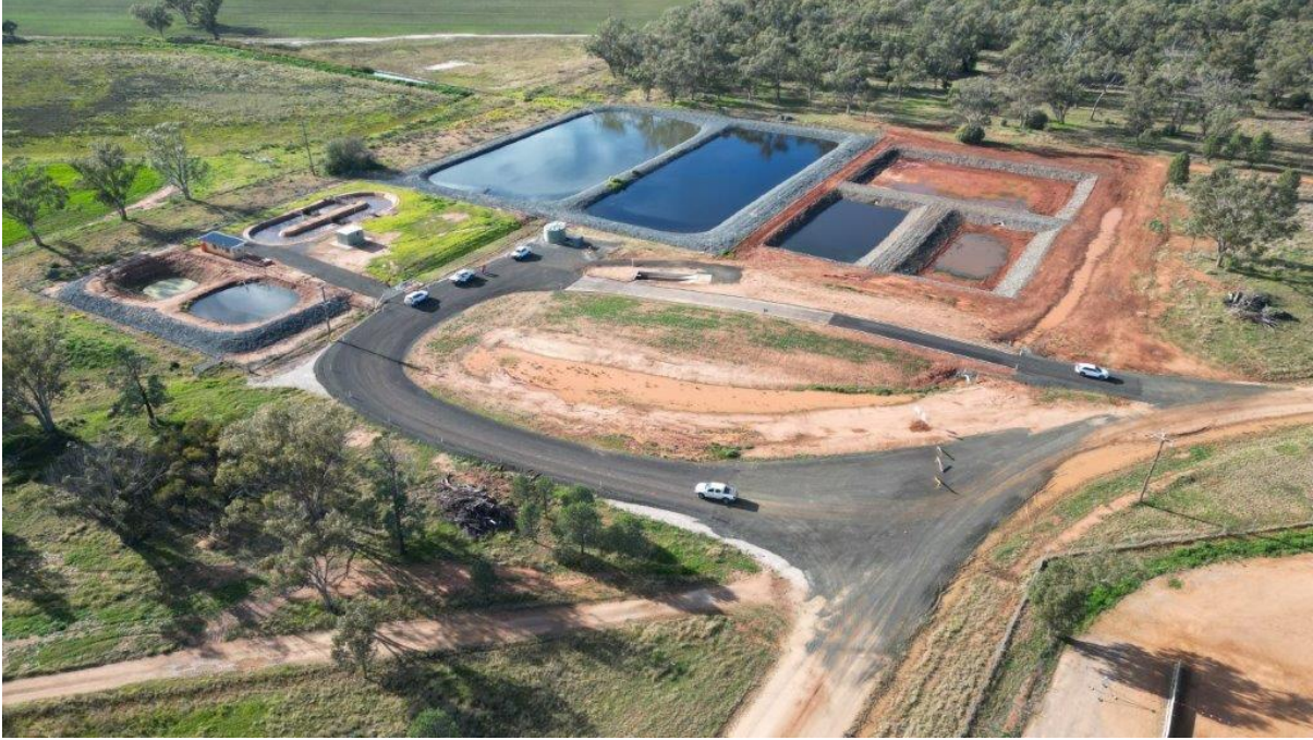
Figure 7: Trangie Truck wash is complete
