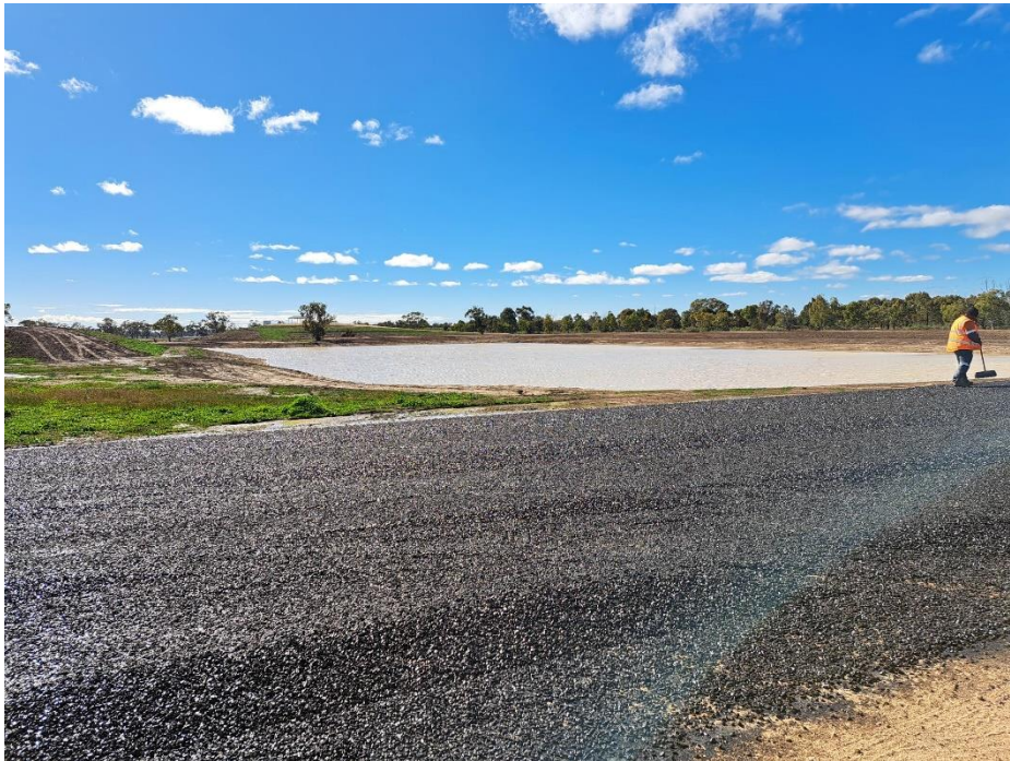
Figure 3: Sealing at the Wetlands Carpark
